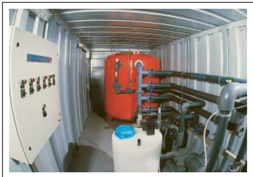
EUROWATER pressure filter built into a container.
