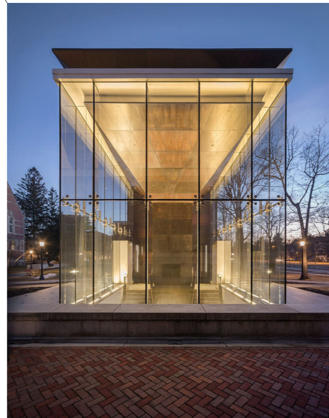
Festive and elegant entrance to the office building
